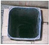
To finish the installation the overhanging pieces of the FURANFLEX® tubes are cut off using a simple saw. Following this the internal thermoplastic foil can be easily removed from the now rigid FURANFLEX®
